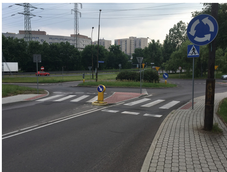
Fig. 3. An example of C-12 sign without sign A-7 on intersection in Sosnowiec, Poland
